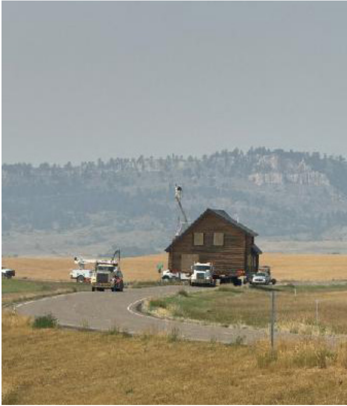
A large home moved through Southeast Electric Cooperative territory at the end of July. Linemen lifted 43 lines in 2 days. | PHOTO BY SARINA O'CONNOR
